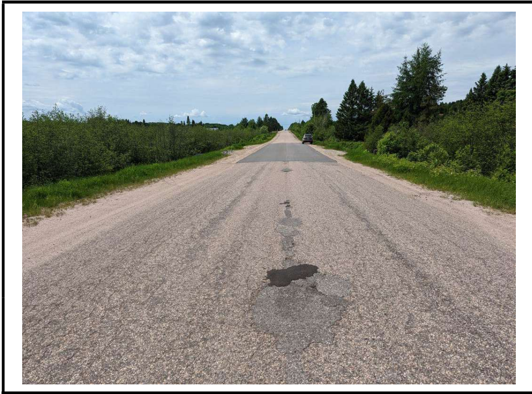
Photo 1 Structure from east approach
