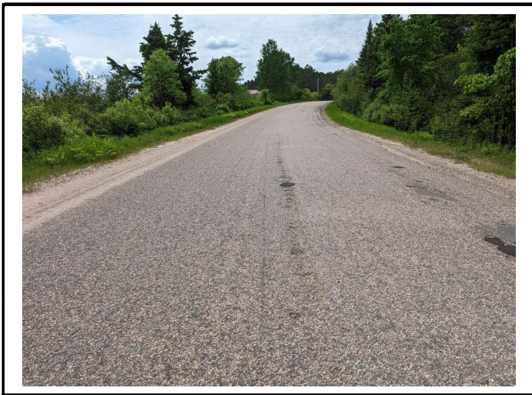
Photo 4 West approach from centre of structure
