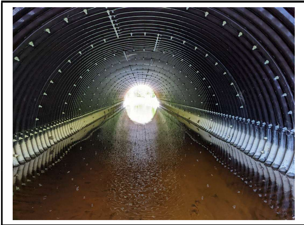
Photo 8 Typical view of culvert barrel looking south
