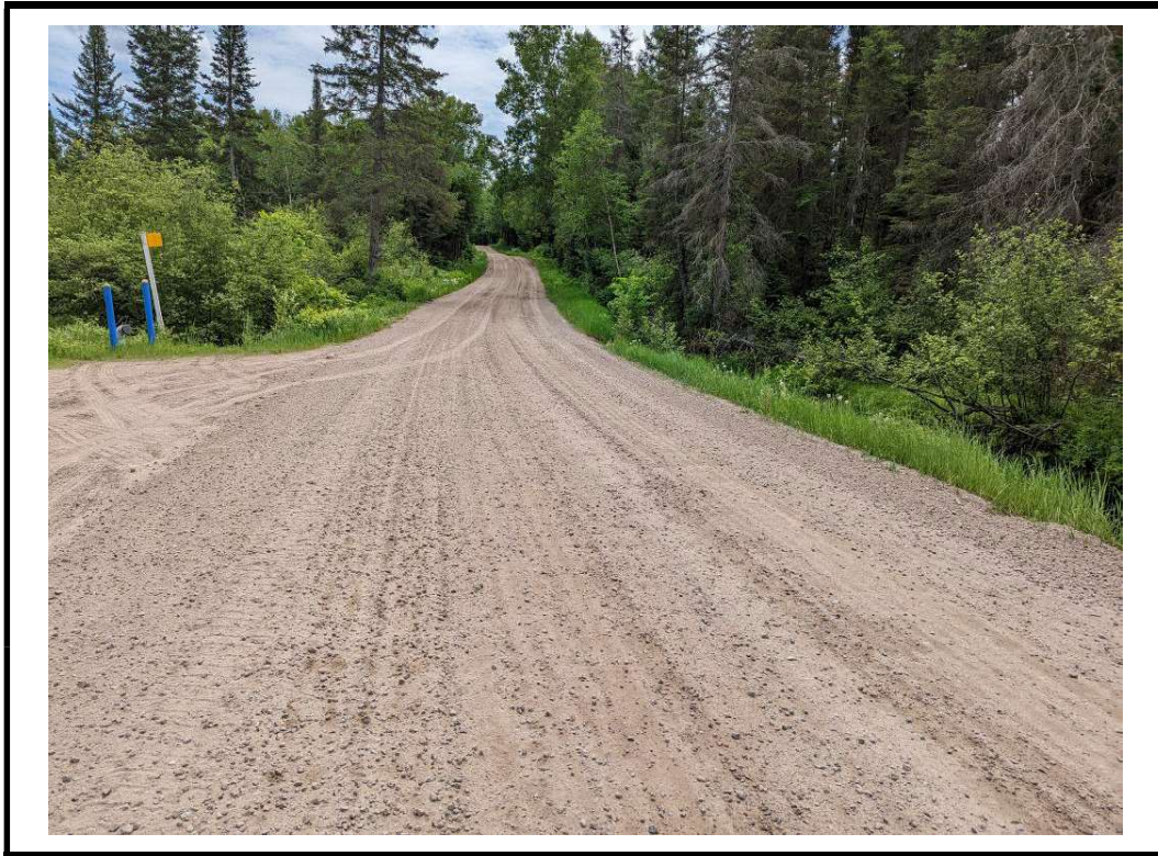
Photo 1 Structure from north approach
