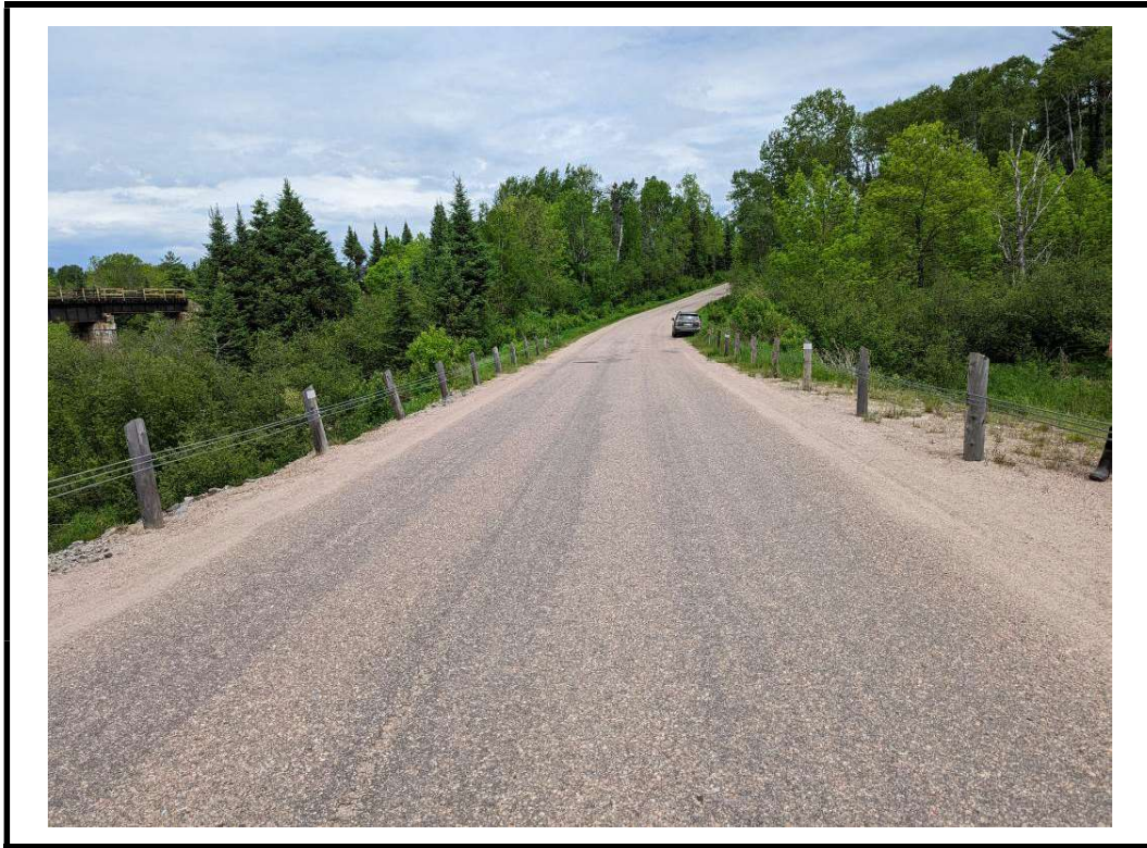
Photo 3 East approach from centre of structure
