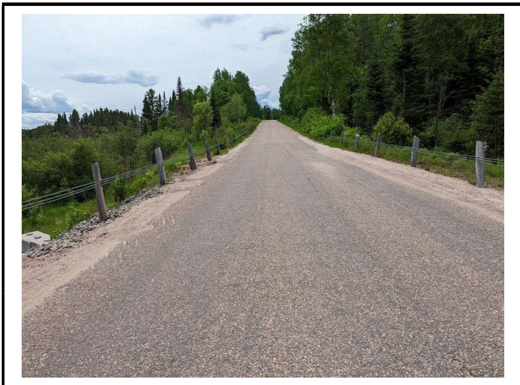
Photo 4 West approach from centre of structure
