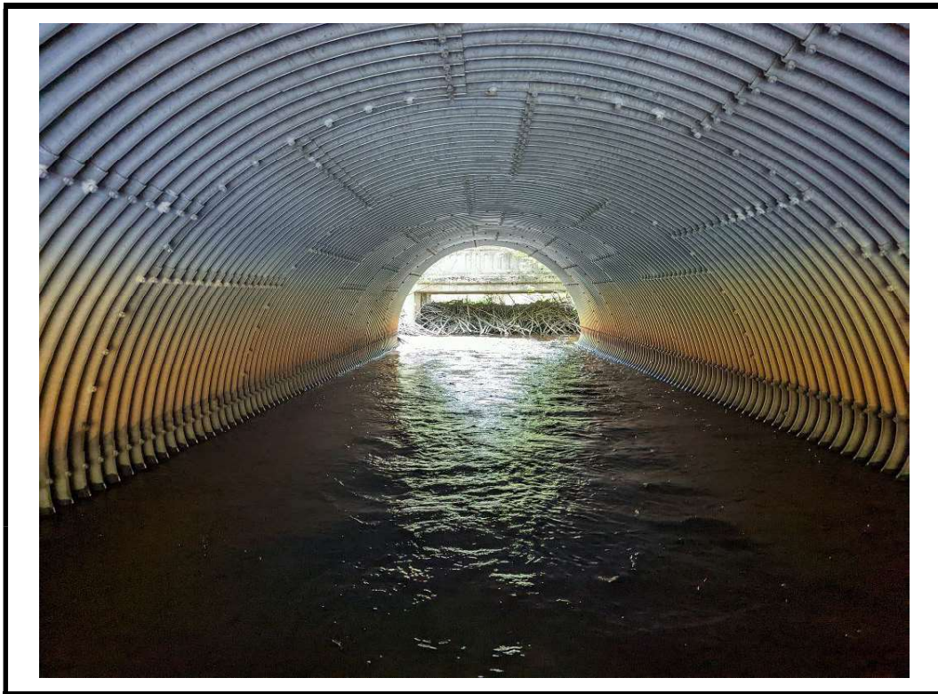
Photo 10 Typical view of culvert barrel looking south
