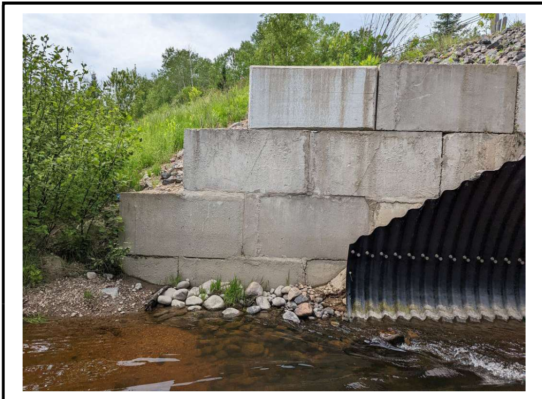
Photo 12 Typical pre-cast concrete block retaining wall at southwest corner of culvert
