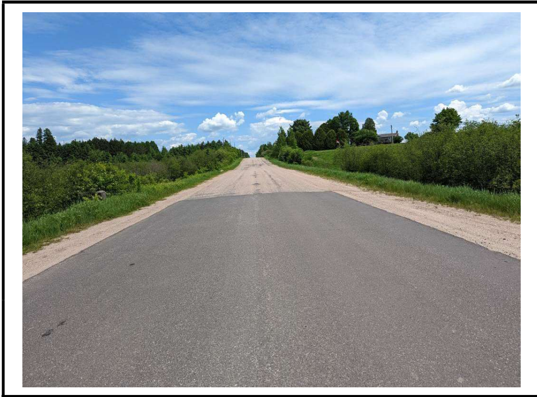
Photo 3 East approach from centre of structure
