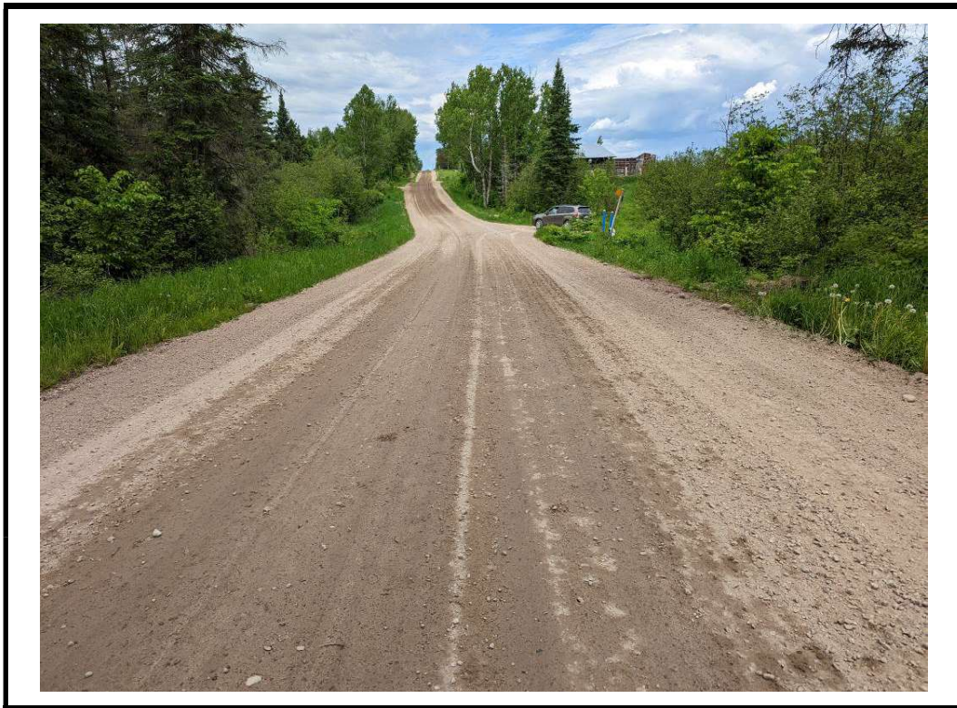
Photo 2 Structure from south approach
