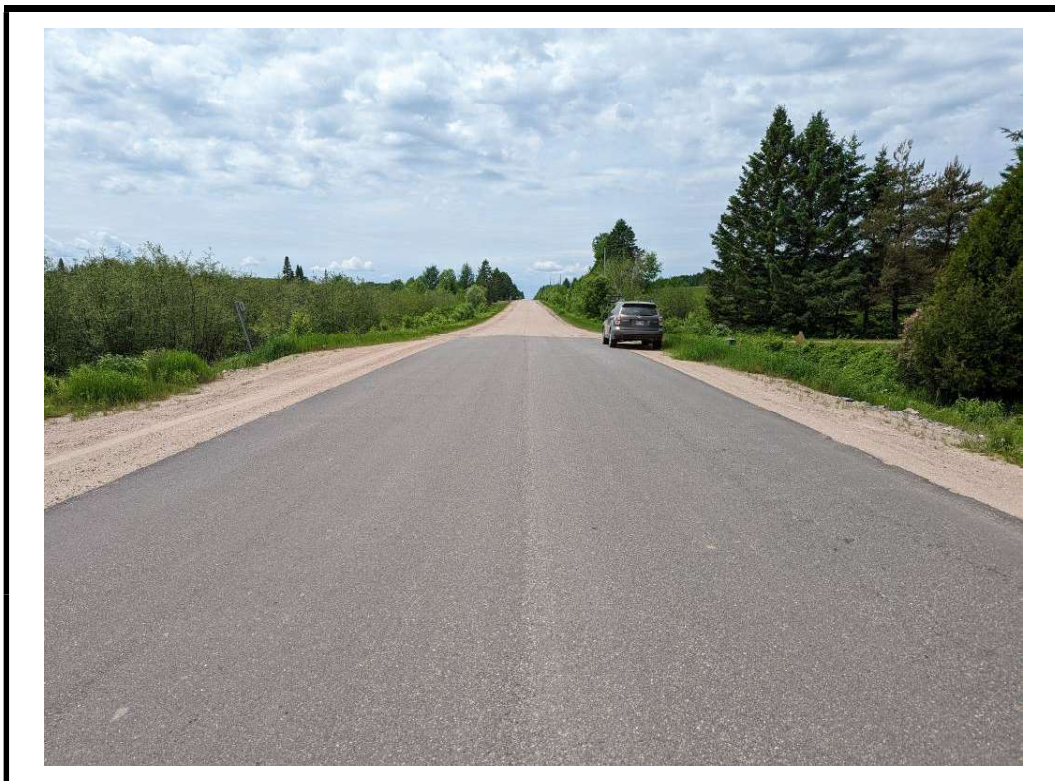
Photo 4 West approach from centre of structure
