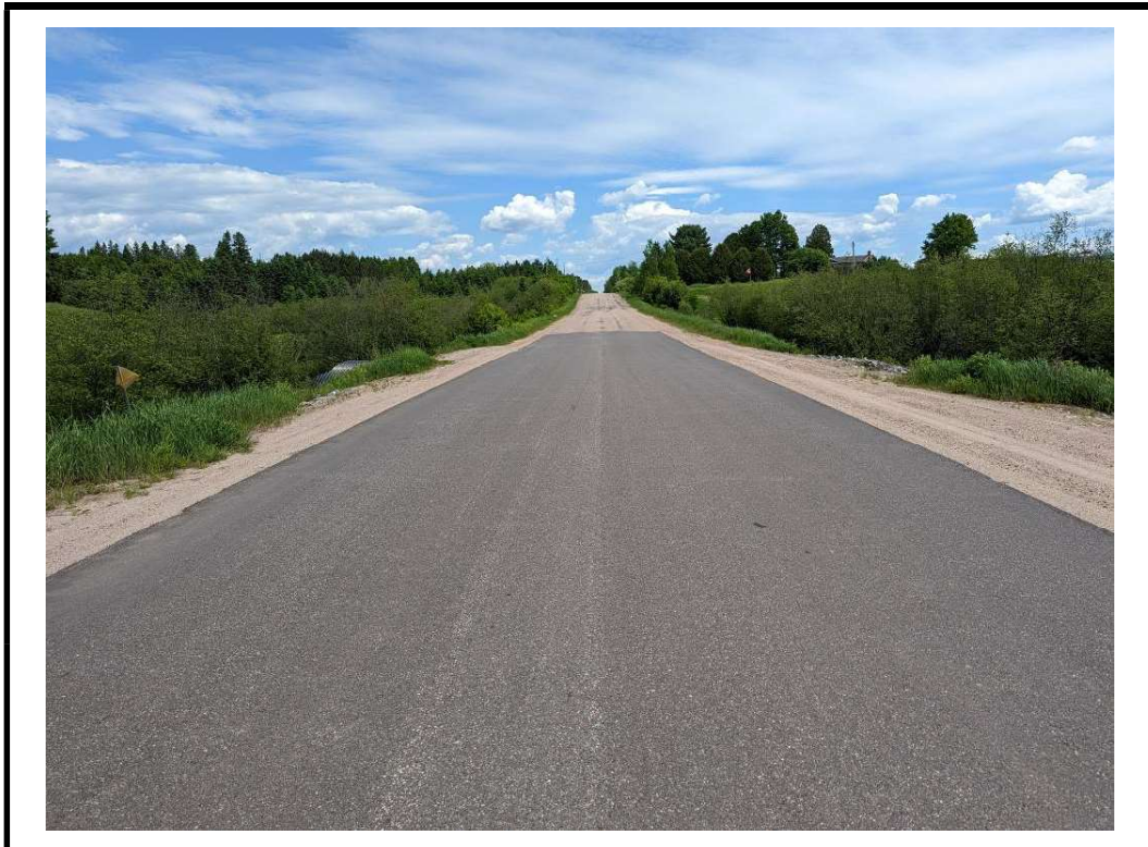
Photo 2 Structure from west approach
