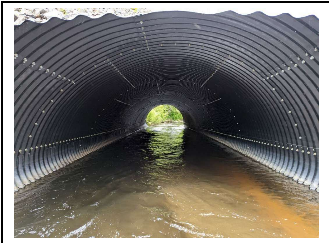
Photo 10 Typical west culvert barrel looking north
