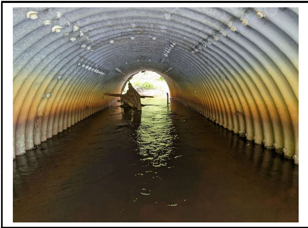
Photo 9 Typical view of culvert barrel looking west
