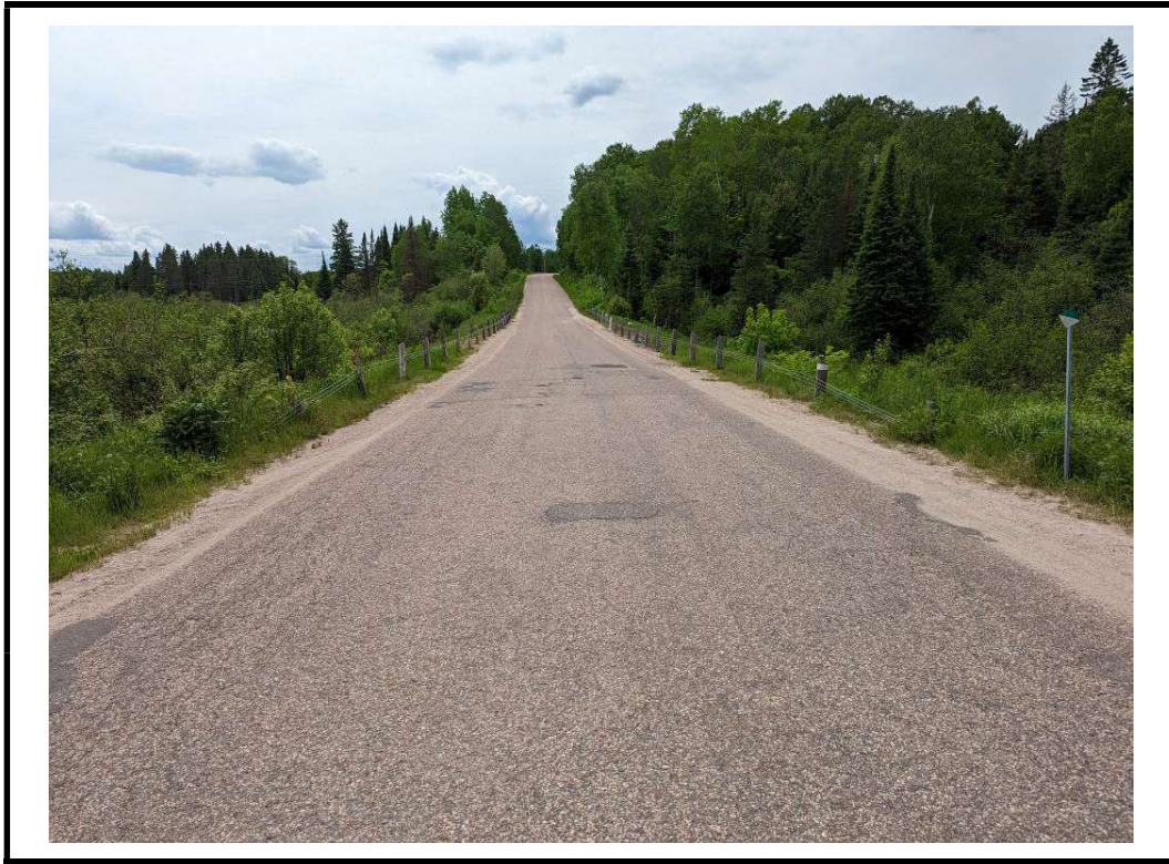
Photo 1 Structure from east approach
