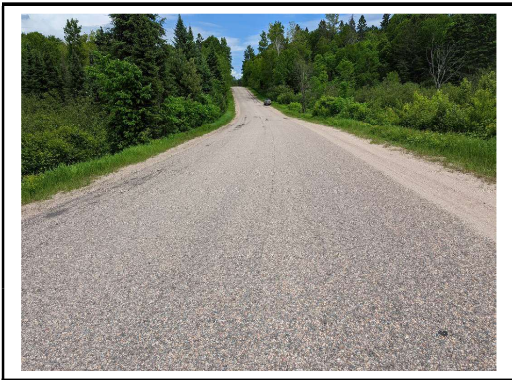
Photo 2 Structure from west approach
