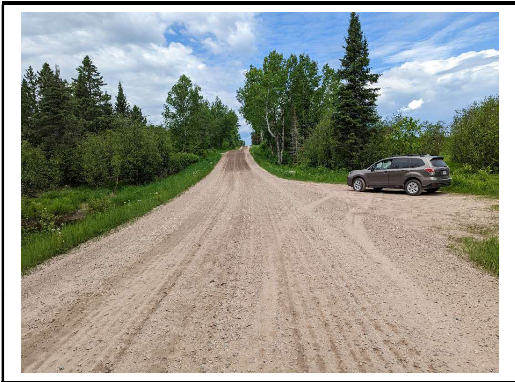
Photo 3 North approach from centre of structure
