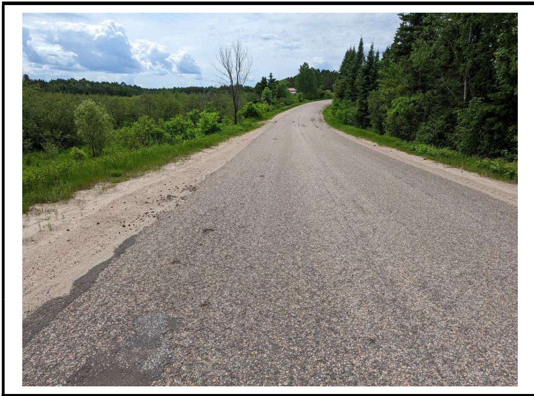
Photo 1 Structure from east approach
