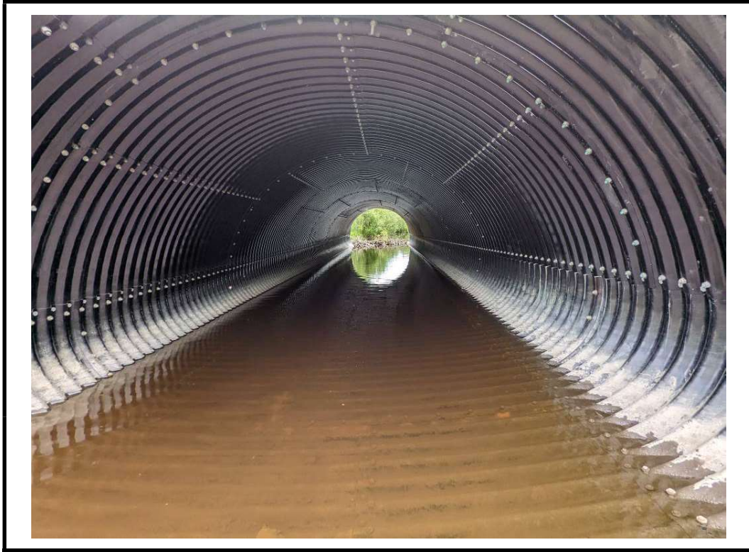
Photo 9 Interior of east culvert barrel looking south
